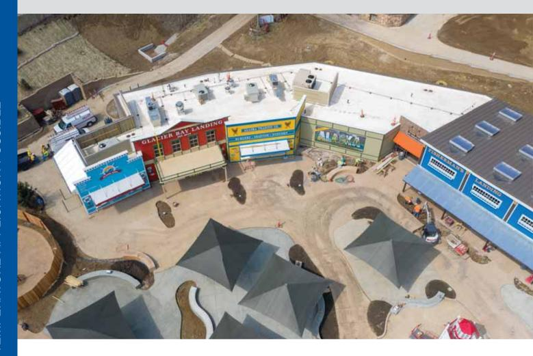
The concession building rooftop also featured two additional layers of polyiso insulation. The initial layer of InsulBase was followed by a layer of tapered polyiso crickets with a half-inchper-foot taper. Like the sweet shop rooftop, the insulation was completed with a layer of Carlisle's InsulBase RL polyiso.
