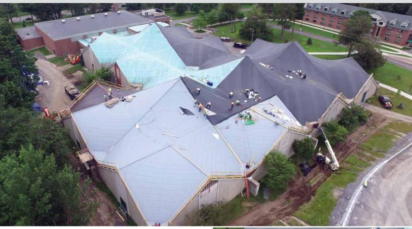
Because of this unique structure, the rooftop material chosen for this re-roofing project needed to be flexible, while also being durable and energy-efficient to protect the building and those inside from the extreme northern winters. With all of these elements in mind, a one-of-a-kind roofing system manufactured by Carlisle SynTec Systems was chosen: Carlisle's FleeceBACK EPDM fully adhered roofing membrane.
