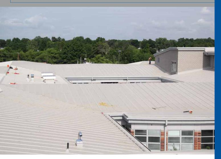
DuPont® Elvaloy® KEE HP, a solid, high-molecular-weight plasticizer that will not migrate out of the membrane over time. KEE HP is extremely durable and its wide window of weldability contributes to a quick, efficient installation process, and the solid nature of the KEE HP minimizes smoke during the welding process and increases the low-temperature flexibility of the
