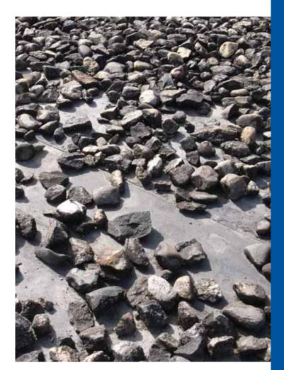
inches of expanded polystyrene (EPS) insulation directly to the metal deck, and then installed the EPDM membrane in 20' x 100' and 45' x 50' sheets. Field-fabricated accessories were used to complete the roof details, and the ballasted system was finished with inch and a half stone loose-laid on top of the membrane.
