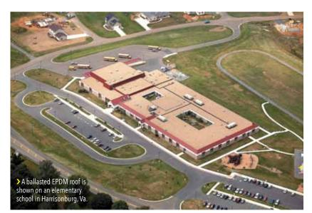
because ballasted systems have something reflective cool roofs don't — the ballast material above the membrane provides thermal mass, which acts as a heat sink and helps protect the building from heat gain. Thermal mass also slows down heat flow, so the heat that does enter the building does so during off-peak hours, when energy costs are often lower.
