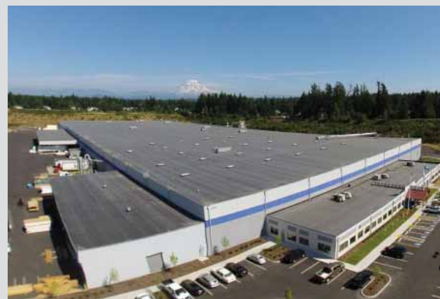
The completed Puyallup, WA insulation plant.
