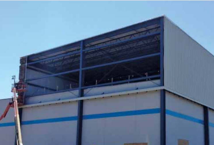
The roof being raised at the Greenville, IL plant.
