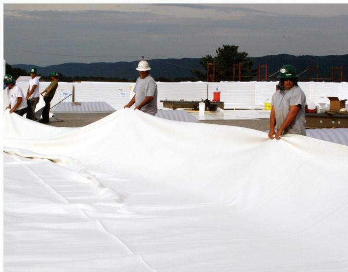
an important aspect of selecting this roofing system, making Carlisle's energy-efficient polyiso insulation and Sure-White EPDM membrane ideal choices for the job.
