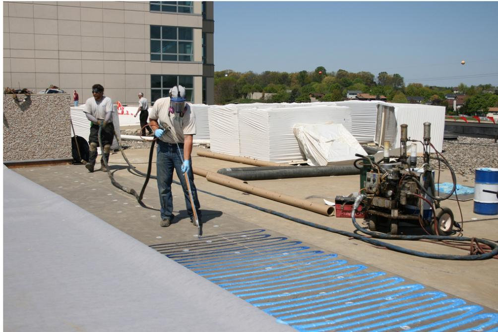
4. **Bead Adhesive Spacing** – Beads must be applied following spacing approved for specific project conditions (i.e. height, wind zone, and warranty wind speed coverage).
