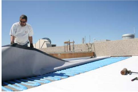
b. Perimeter bead spacing is typically at 6-inches on-center except for those projects with higher wind speed coverage where narrower bead spacing of 4-inches on-center may be required.
