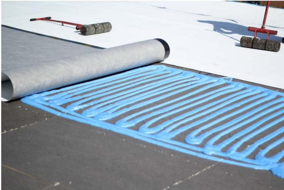
3. Allow the adhesive to rise up approximately 1/4" and develop string-time prior to setting insulation boards into adhesive.
